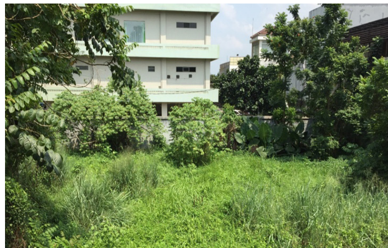
Photo 01. Abandoned Building of GKI Taman Yasmin Bogor
